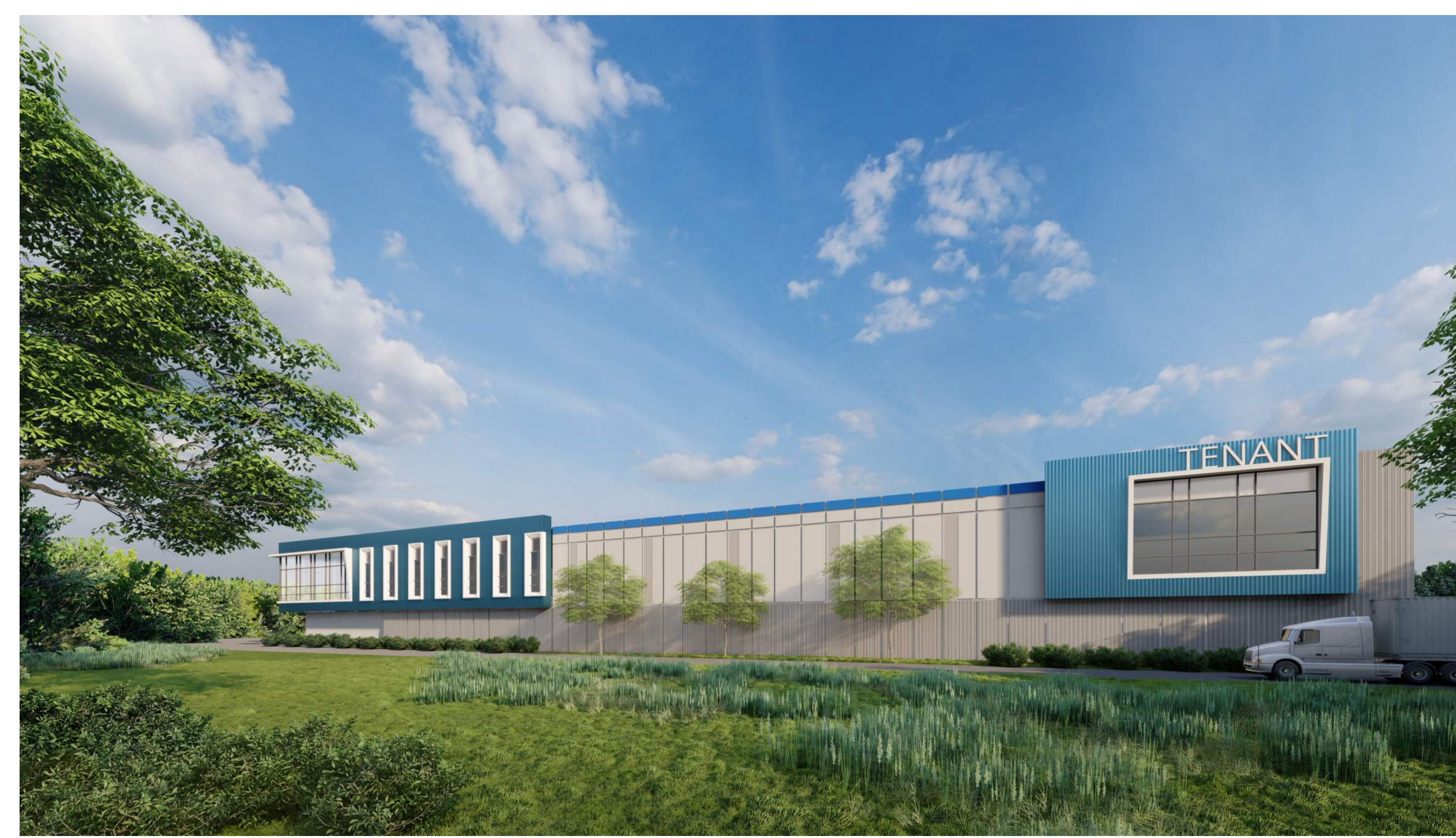
VIEW OF NORTH ELEVATION (FACING I-95)
